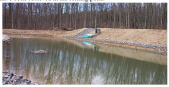
The North Branch Robbins Hollow passive treatment system has been successfully treating AMD with high acidity, high aluminum, and high iron since going online in 2004. Maintenance in the form of replenishing the organic compost (with limestone fines) and washing the limestone in the two vertical flow ponds was conducted in 2012 as preventative maintenance to ensure the continued performance of the system.
