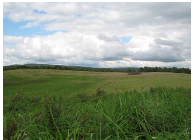
Regrading, addition of organic and alkaline amendments, and establishment of vegetation at the Twomile Run surface reclamation project has resulted in a reduction of 30-40% of the AMD pollution from this area to Twomile Run.
