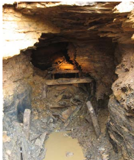
A glimpse into the past: Excavations in the Middle Branch watershed uncovered this deep mine entry. Black coal is visible on left side of picture and wooden posts show where the haulage way once existed.
