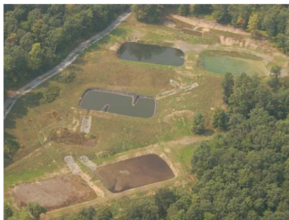
Aerial view of the Middle Branch Passive treatment system. Photo provided by A. Wolfe
