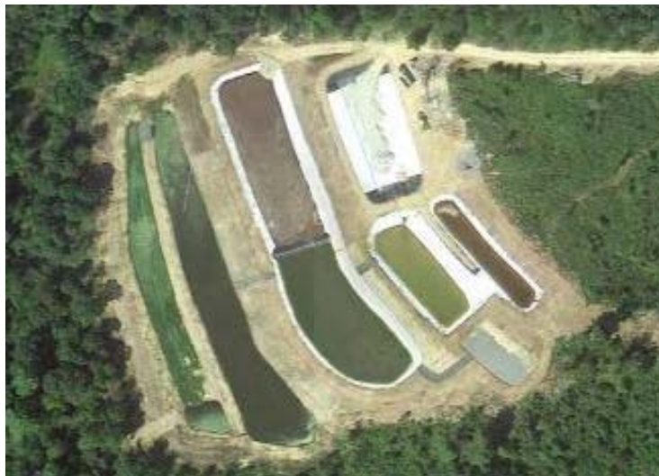
Aerial view of Swamp Area passive treatment system from Google Earth.
