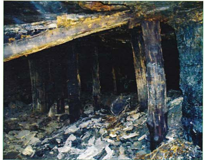
Glimpse into the Past - view looking into the deep mine when the collapsed mine entry was opened (was later backfilled and closed); can see that the roof and pillars are still in relatively good condition; Kettle Creek Coal Company started mining here in the late 1880's until they went out business with the stock market crash in 1929.
