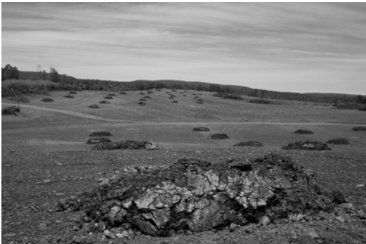
Piles of WesTan soil on the abandoned mine site await spreading and mixing into the top 6 to 10 inches of surface material which consists primarily of shale and sandstone.
