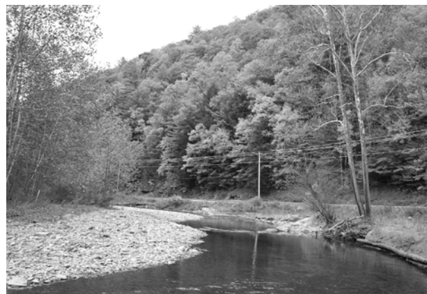
Looking downstream at the Headgate project (State Route 144 on right). Picture taken in mid-October 2004, approximately one month after Ivan.
