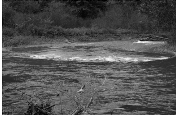
Looking downstream at Kettle on upper end of Delayed Harvest Special Regulations project site. Notice how the cross vane diverts flow away from streambanks.
