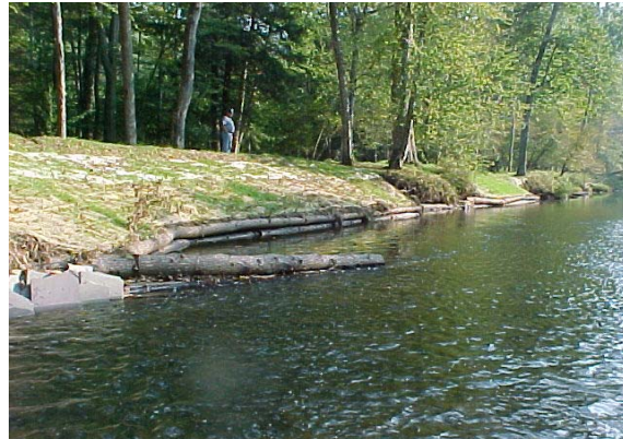
Completed mud sills and log vanes provided immediate cover from hot summer sun for the trout.
