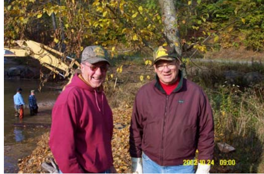
This project would not have been as successful without the commitment of KCWA volunteers. Pictured here are Al Lyons (left, KCWA member) and John Larson (right, KCWA President). Special thanks to John for his long hours at the project site nearly every day!
