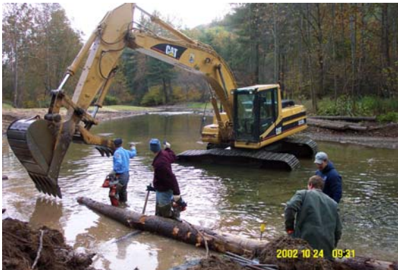
Dave Keller (Habitat Management Section Manager for PA Fish & Boat Commission) and George Daniel (PA Fish & Boat Commission) give the equipment operator, Don Stover of the USFWS directions for moving the logs during installation of the mud sill. Neil Wolfe (KCWA/TU) and Jared Dressler (USFWS) are standing to the far right.
