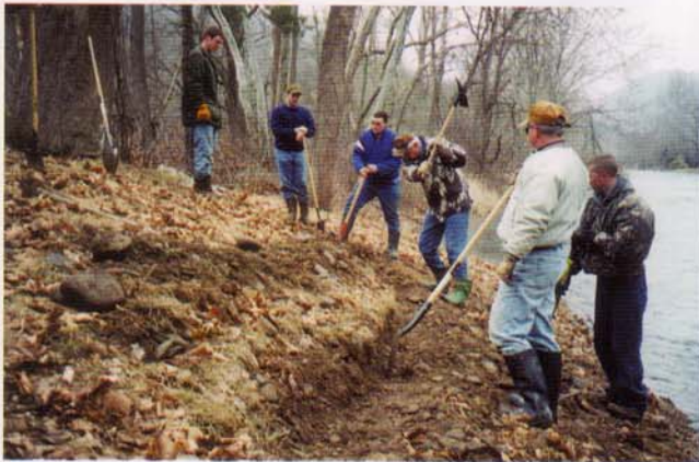
A terrace is dug on the regraded streambank for brush layering.
