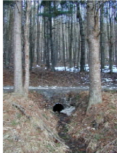
Small culvert at Ole Bull State Park.
