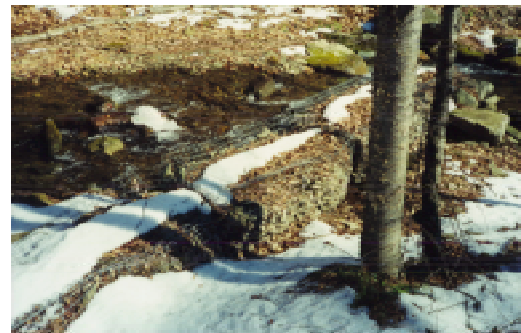
Gabion on Elk Lick Run
