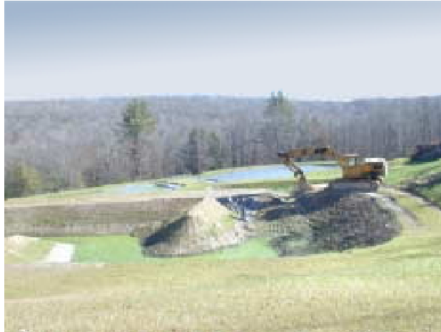
AMD remediation on the Kettle Creek watershed
