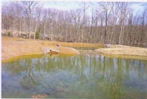
Side-by-side vertical flow ponds containing mushroom compost and limestone treat mine drainage discharges in Robbins Hollow.
