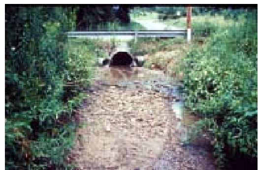
Figures 5.16, 5.17 - Road crossings can be the single largest contributor of sediment to a stream on forested watersheds. Additionally, road crossings can limit fish passage, cause localized erosion and be a costly maintenance problem after floods. Stream crossings are listed by subwatershed in the chart above for comparison.
