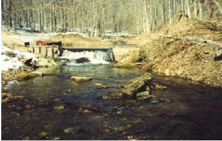
Small dam located on Elk Lick Run
