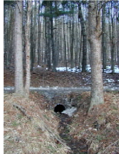
Small culvert at Ole Bull State Park.
