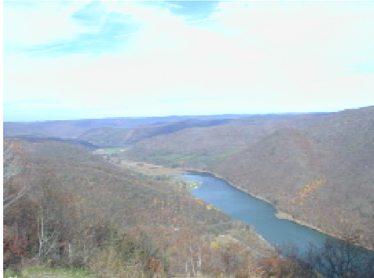
The Alvin R. Bush Dam was designed to control floodwaters in the West Branch and created this reservoir in Kettle Creek State Park.
