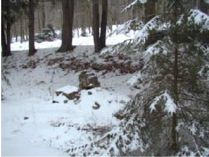
A snow covered foundation of a cabin built by the Civilian Conservation Corps Camp S-87 in Ole Bull State Park.
