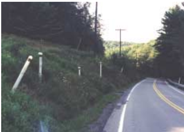
The natural gas pipelines impact both the environmental integrity and the scenic quality of the watershed by cutting through the forested hillsides.
