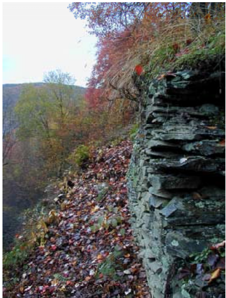
A portion of the Ole Bull Castle's foundation in Ole Bull State Park.
